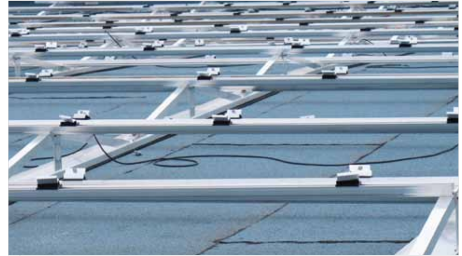
Frankental | Germany System: 58 kW | D-Level System
